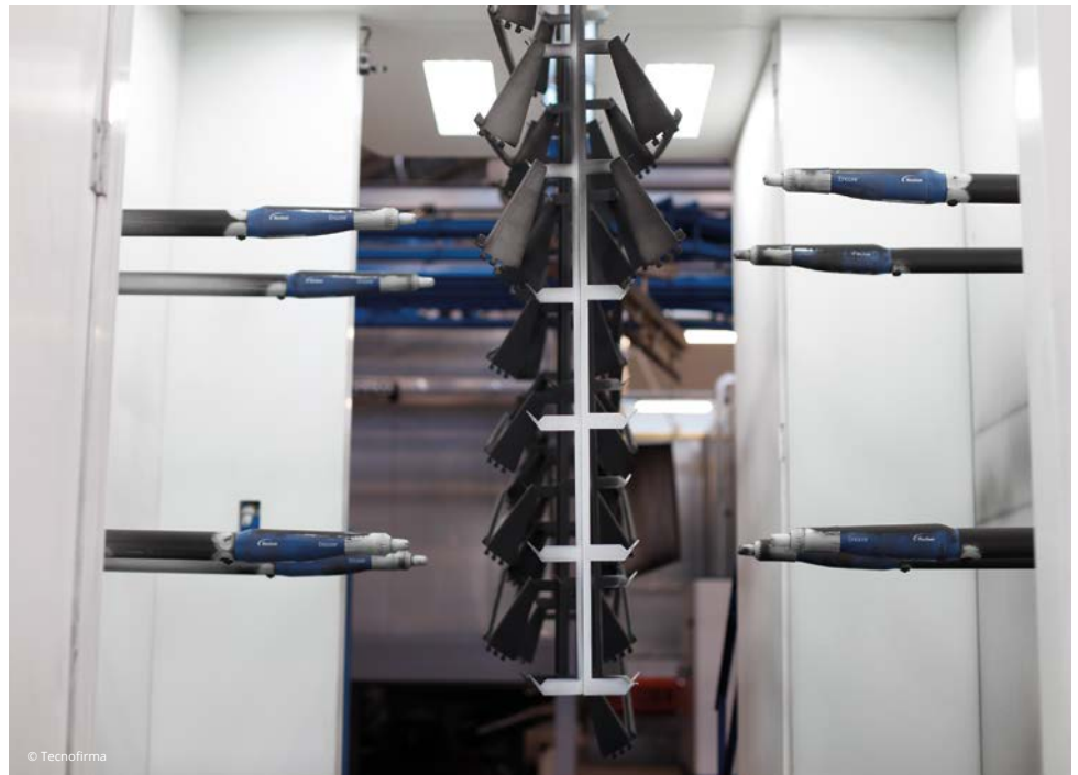
Interior of the coating booth.
