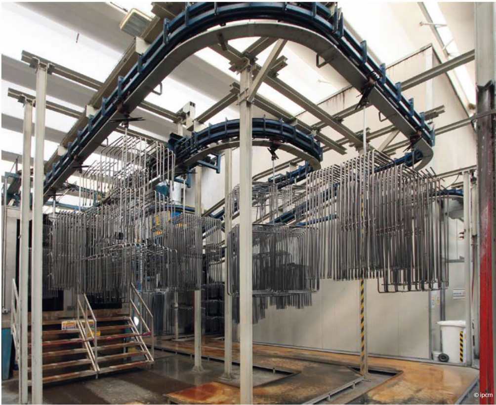
The pre-treatment tunnel.
