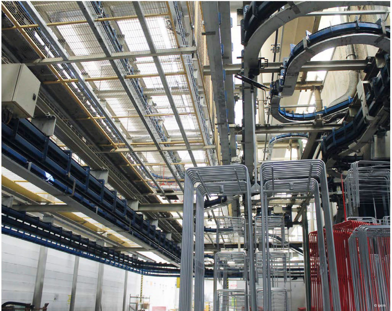
A segment of the conveyor.
