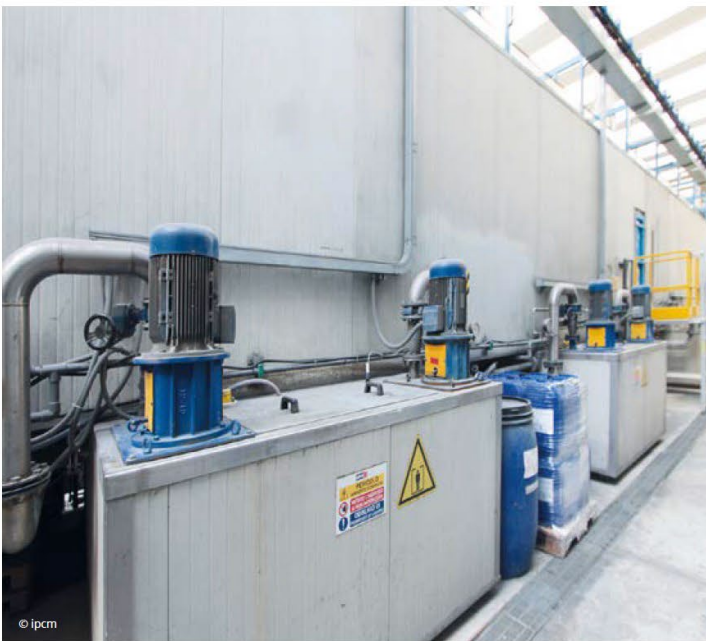
The outside of the pre-treatment tunnel.
